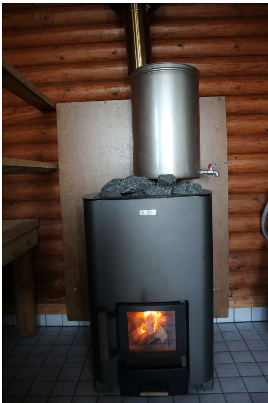
Figure 1.6. Sauna stove with a hot water tank (Tykkyläinen, 2019).
